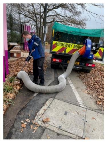
With additional help from our Street Cleaning team we're able to keep the wider pathways clear using our <u>Hako</u> Sweeper. We are also now equipped with a Terrier T10 Leaf Vacuum, which mulches the leaves so we're able to collect more are one time.
